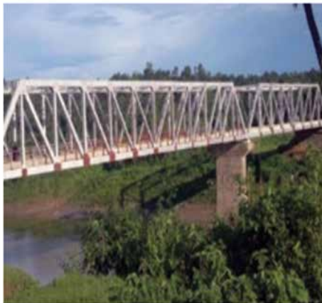
RCC Bridge over River Dholeswari
